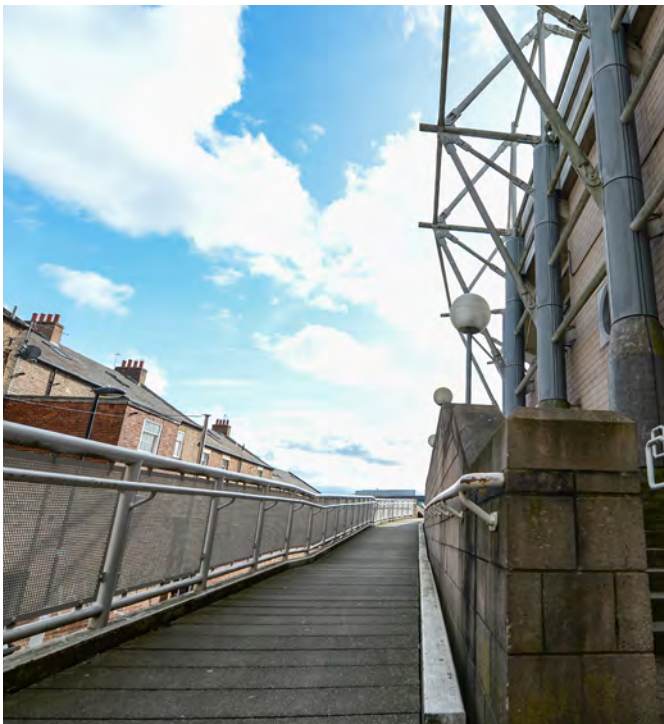
Figure 12. Access ramp located in the South East corner
