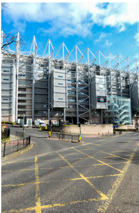
Figure 4. Access to the Stadium Car Parks via Barrack Road
