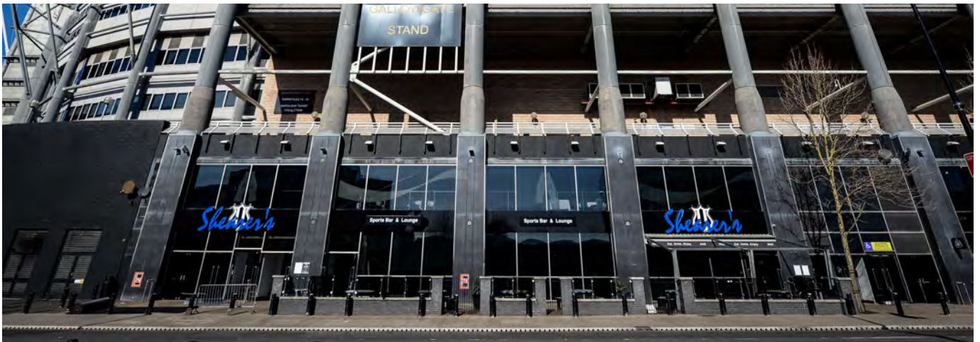
Figure 23. Ramp into “Shearer's Sports Bar’ with assisted entry doors
